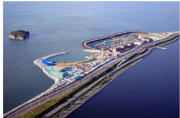
Figure 7. A view of Sihwa Lake Tidal Barrage (Bae et al., 2010).
