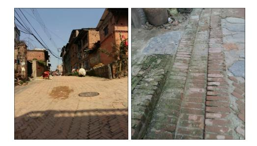
Figure 4. Street and brick paved drain in Bhaktapur in 2017, Source: The Author
