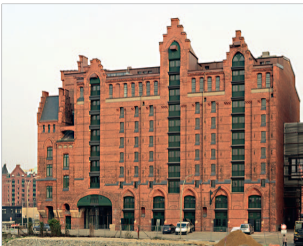
Fig. 9. Historic building reconstruction in Hamburg
