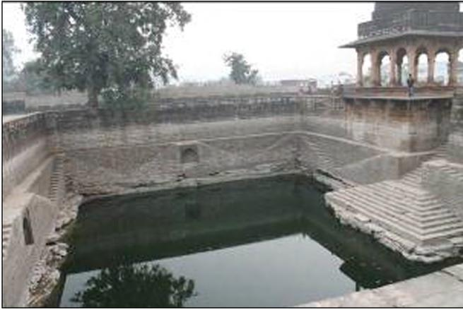
**Figure 9** View of the rectangular stepped pond showing the niches in the walls and triangular formation of steps to access water. Image Source: Author during field visit.
