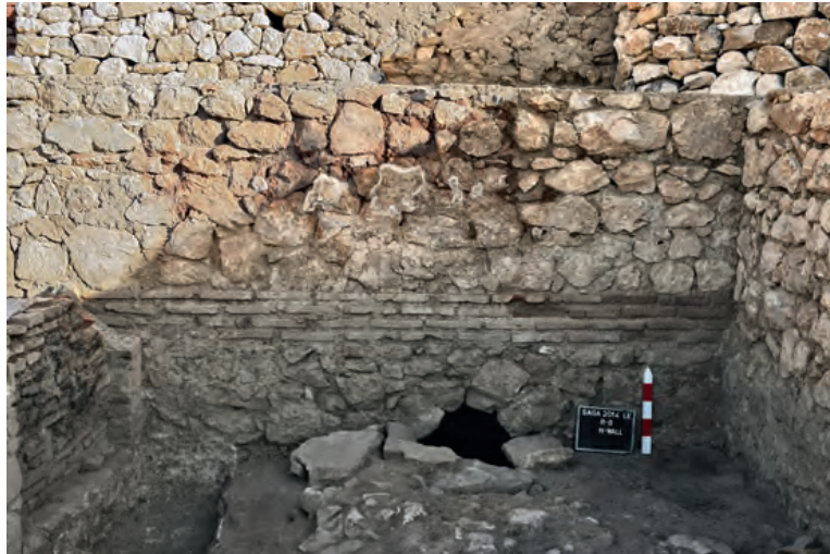
Fig. 6. Opus vittatum as used in the unidentified public building.
