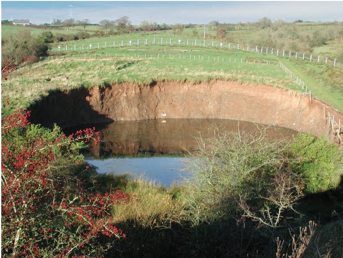
Figure 11. Maidenmount Salt Mine near Carrickfergus which collapsed on 19 th August 2001 and was initially 50 metres wide and 15 metres deep, but continued expanding (BGS photograph P543378)
