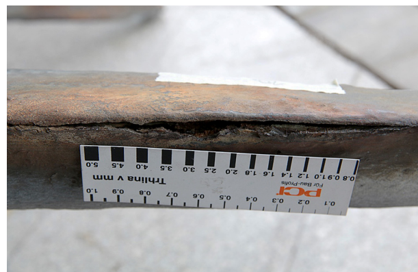
Obr. 3. Prasklina v celé tloušťce laminátu Fig. 3. Crack in the whole thickness of the laminate
