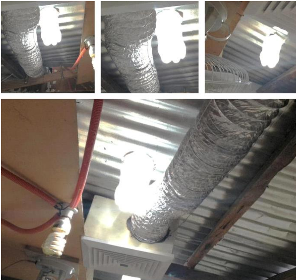
Figure 3. Solar bottle bulbs attached on the roof provide lighting during day time (Mifunedumaguete.com, 2014)
