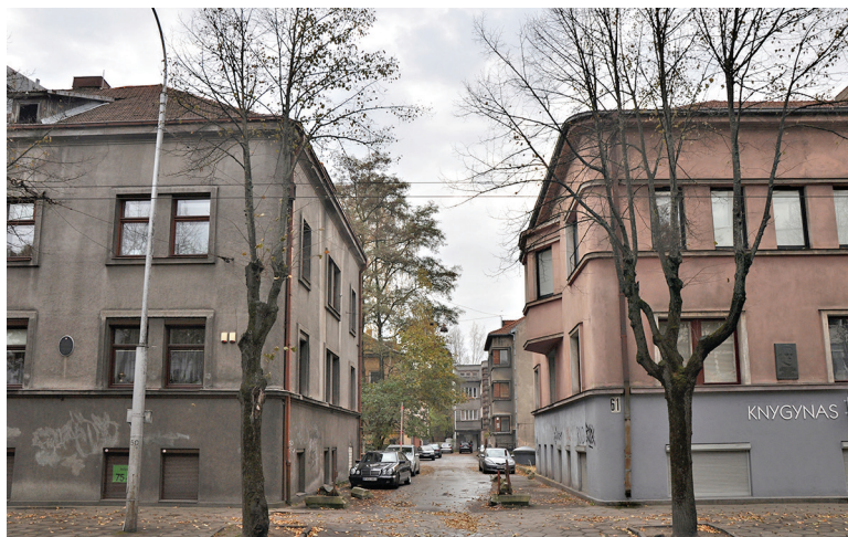
Fig. 3. Residential houses listed as objects containing valuable features in Kaunas downtown area. Photo by V. Petrulis
