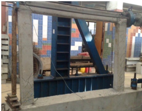
Figure 3. Mode of failure of F1
