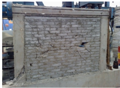
Figure 6. Mode of failure of F4
