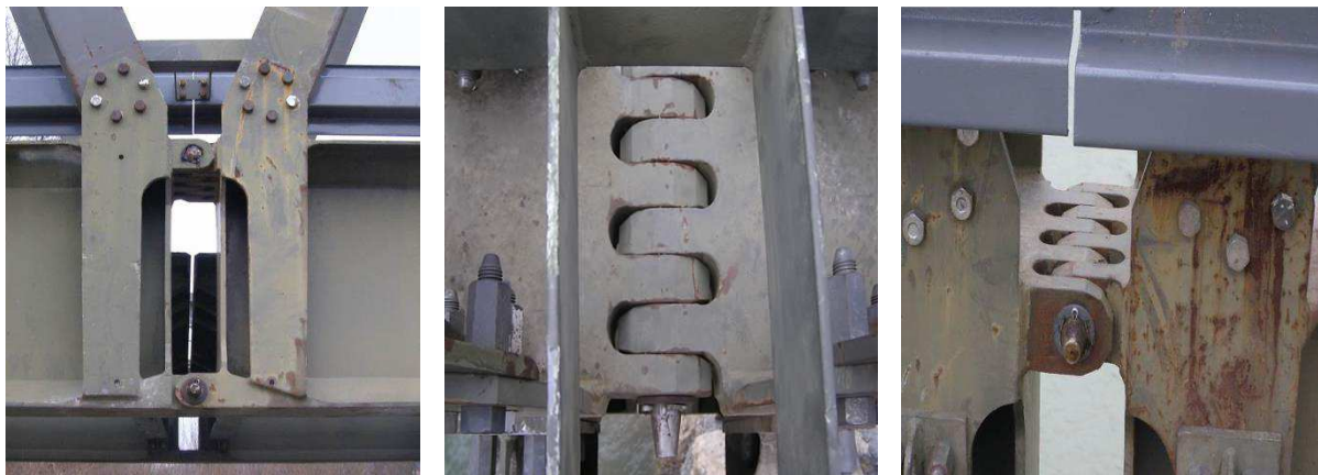
Fig. 1: Pin connection (lock) of the lower chord of the bridge ŽM 60.
