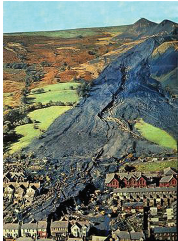
Fig. 1.3. Aberfan in the days immediately after the disaster, showing the extent of the spoil slip ( https://en.wikipedia.org/w/index.php?curid=54882575 ).
