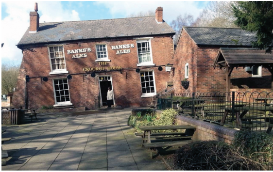
Fig. 1.16. The Crooked House, Dudley, suffering from coal mining subsidence.
