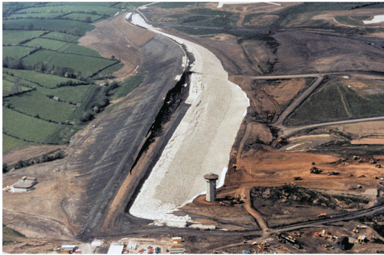
Fig. 1.9. Carsington embankment under construction in 1984 (photo credit: Winter et al. 2017 ).
