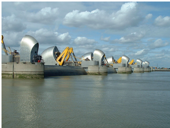
Fig. 1.18. Thames Barrier, London (photo credit: Andy Roberts).
