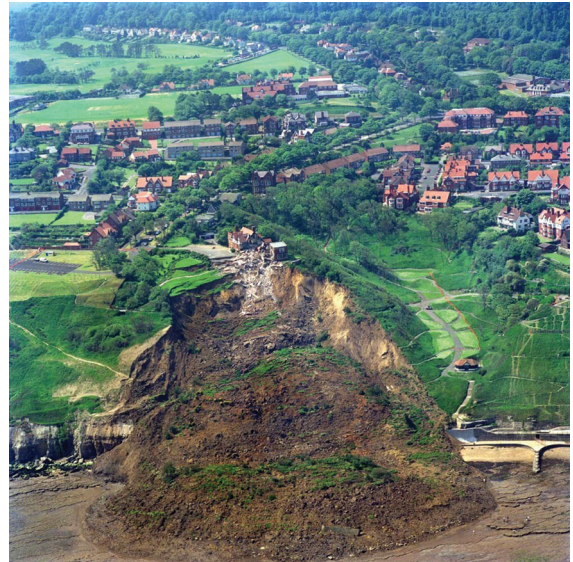
Fig. 1.8. Landslide at Holbeck Hall, Scarborough, Yorkshire, 1983 (photo credit: British Geological Survey).
