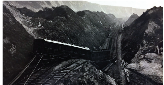
Fig. 1.7. Landslide at Folkestone Warren, Kent, 1914 (photo credit: Network Rail).
