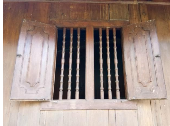
Figure 3. The windows of Pyramid House in Palembang (Documentation: Ario)
