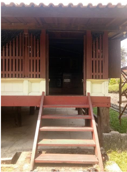
Figure 5. Stairs at Pyramid House in Palembang (Documentation: Rio)
