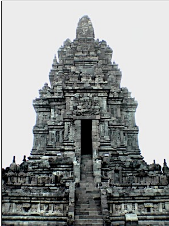
Figure 3. One of the temples at Candi Prambanan, still erect with minor damage, after the 6.4 magnitude earthquake in the year of 2006 (Source: Author Documentation, 2007)
