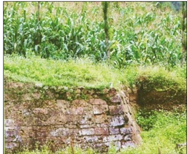
Figure 4. Talud made from tuff square stones (Source: Riyanto, 2018)
