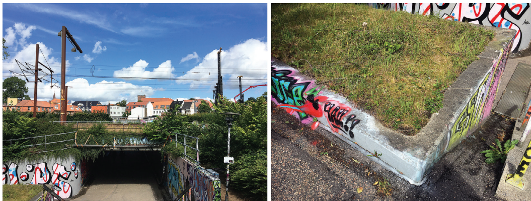
Figure 9: Photo documentation of Site 2 'Graffiti Tunnel' before intervention.
